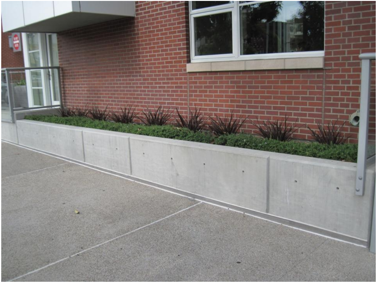
Figure A.5-1. Flow-through planter.
